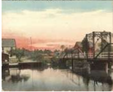
After the ferry, the first swing bridge
